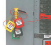
4. For group lockouts, run key through multiple loops in lock rail and apply locks. No hasps required! (Not recommended for use with multilock hasps)
