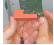
2. Attach the lockout device to the breaker and snap into locked position.
